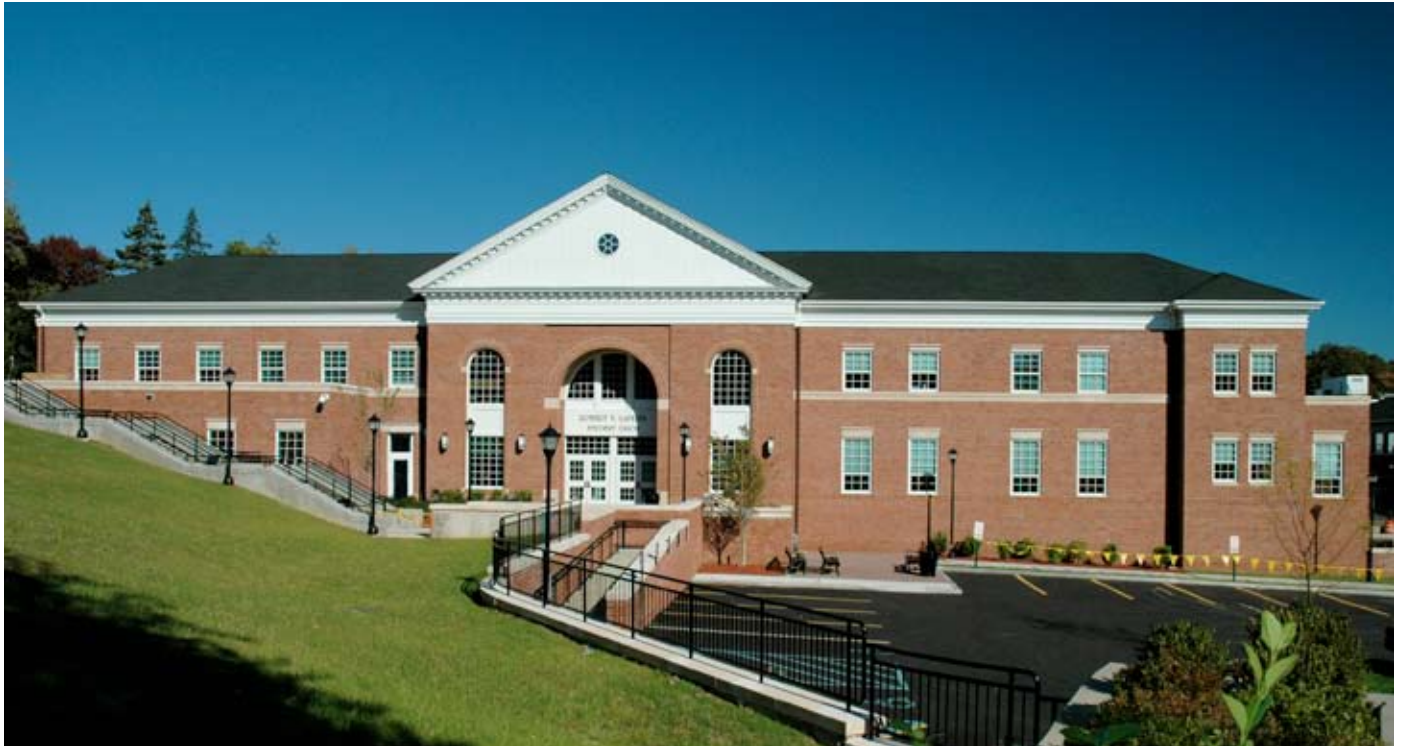
ARCHITECT: Anthony M. Pucillo, Architects Design and photography: RonDubeDesign.com
